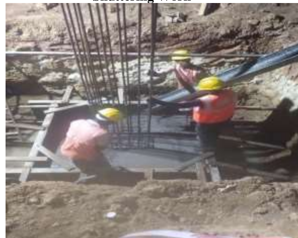
Footing Concrete Work, Pedestal Barbending & Shuttering
