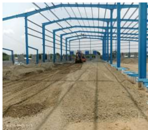
GSB Levelling and Compaction
