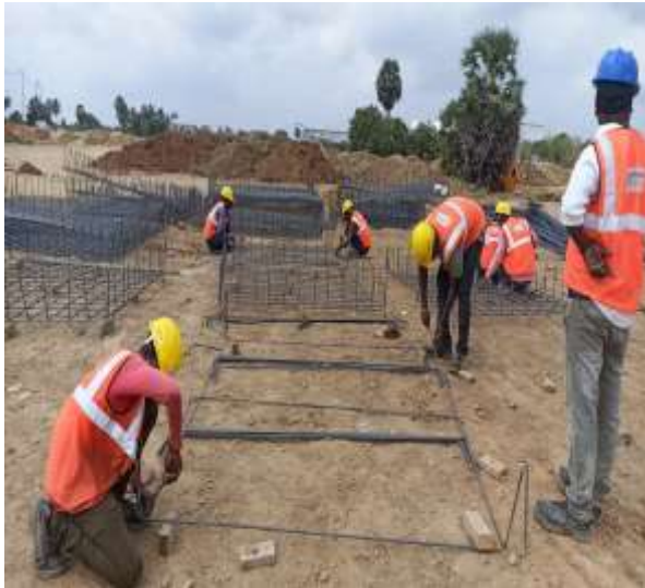
Reinforcement Work
