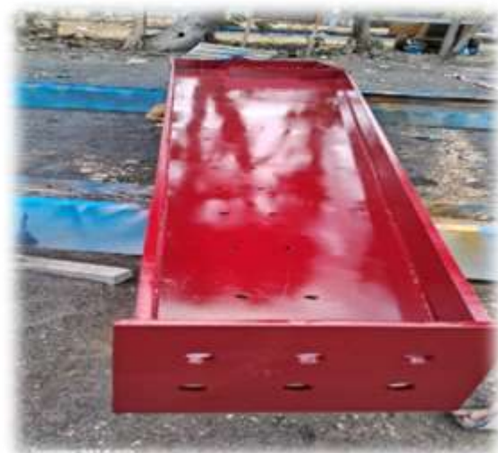
MS Structure Painting
