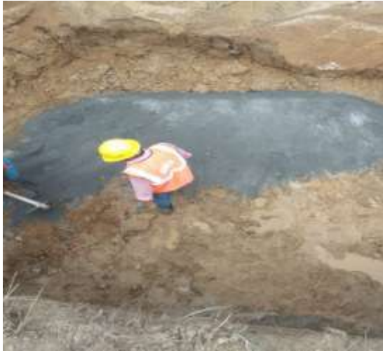
M- Sand Filling Work
