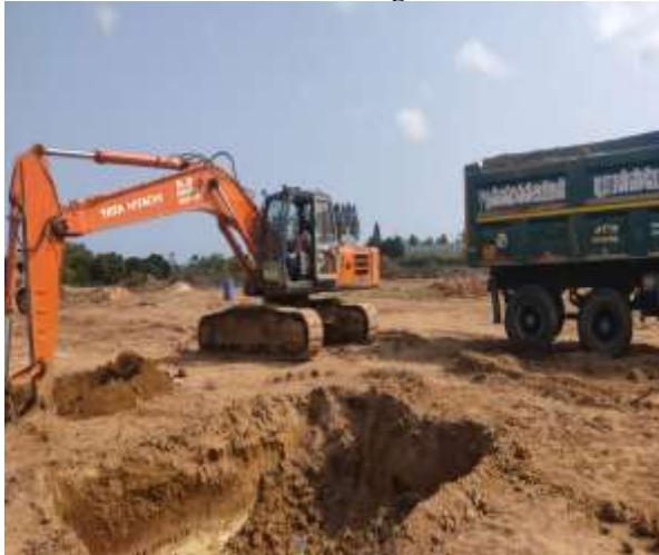
Earth work Excavation
