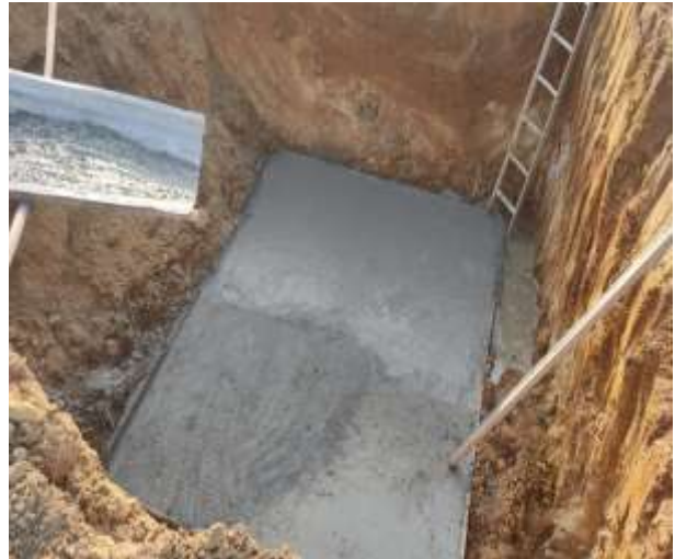
PCC Concrete Work
