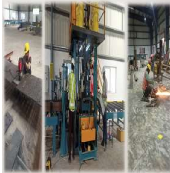
Civil Foundation Fabrication Work
