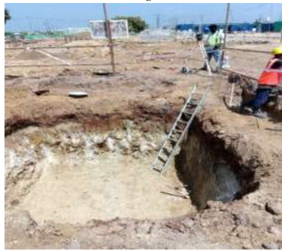
Footing Levelling and PCC Marking Work
