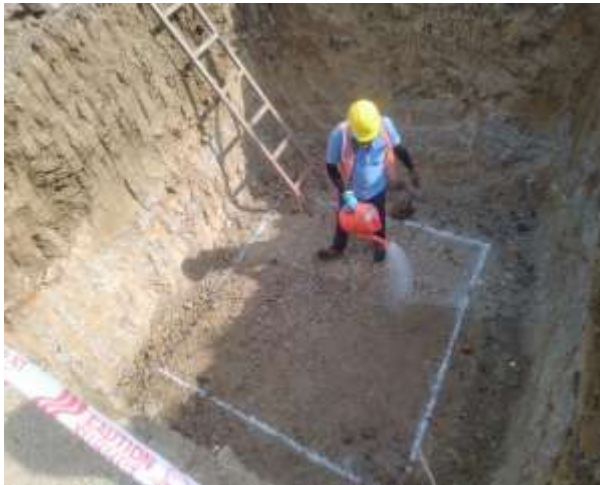
Anti Termite Work
