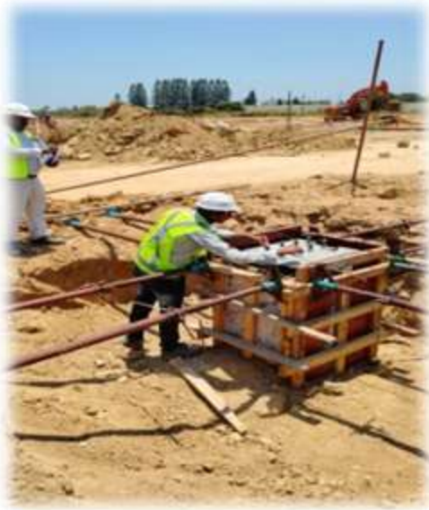
Anchor Bolt Fixing & Checking
