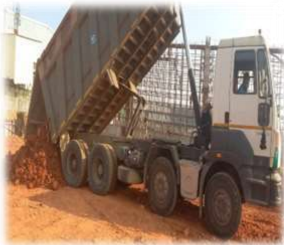
Soil Filling and Compaction
