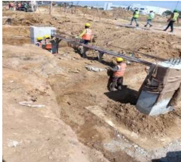
Plinth Beam Shuttering and Concrete Casting
