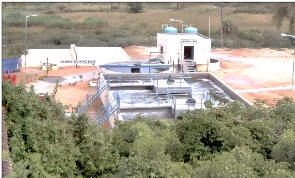
Overview of Sewage Treatment Plant
