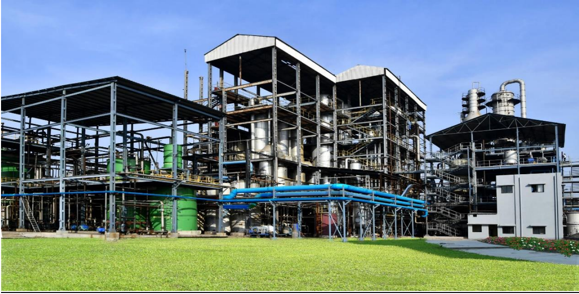
Cogeneration Plant at the Sameerwadi Manufacturing Facility
