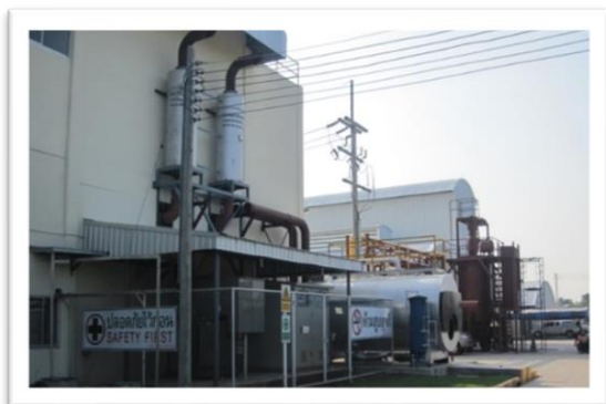
Biomass Power Plant- Satake International, Thailand
