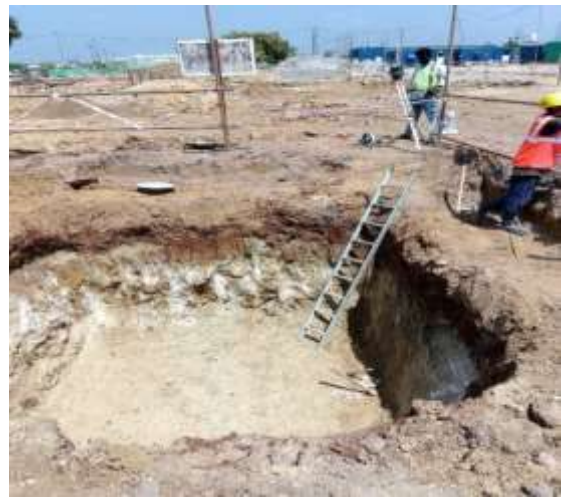
Footing Levelling and PCC Marking Work
