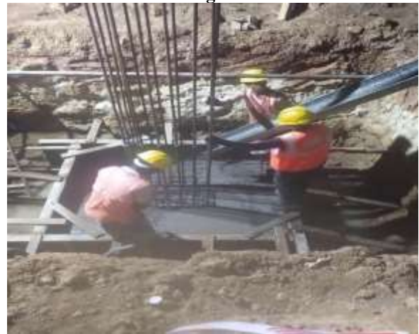
Footing Concrete Work, Pedestal Barbending & Shuttering
