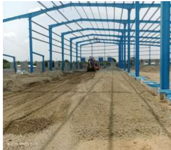
GSB Levelling and Compaction
