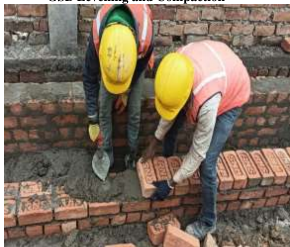
Brick/ Block Work
