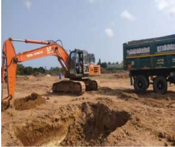
Earth work Excavation
