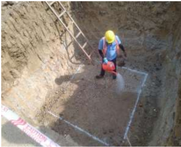
Anti Termite Work
