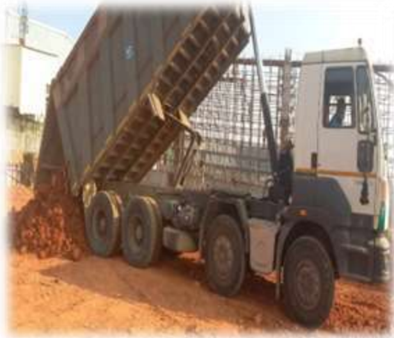
Soil Filling and Compaction
