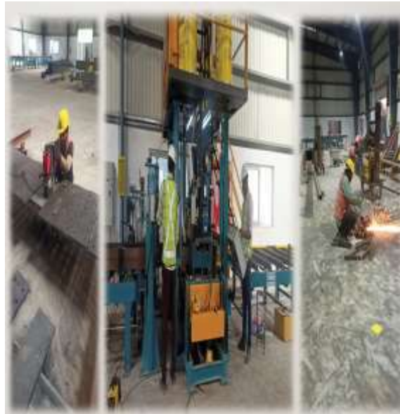
Civil Foundation Fabrication Work
