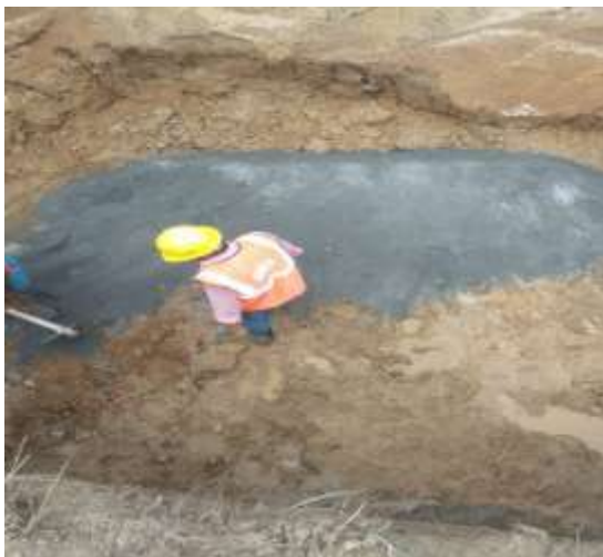
M- Sand Filling Work
