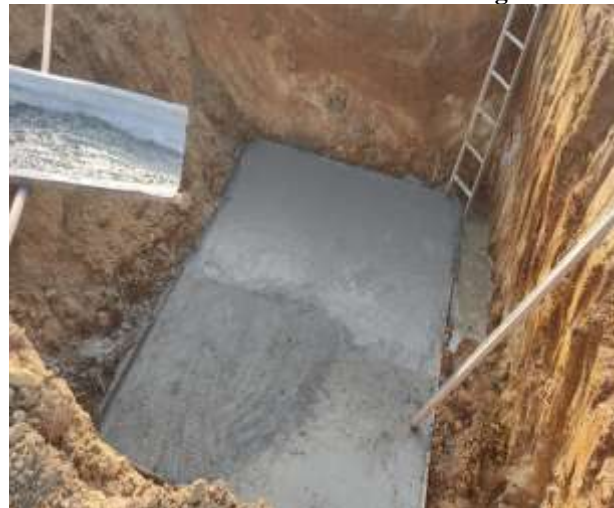
PCC Concrete Work
