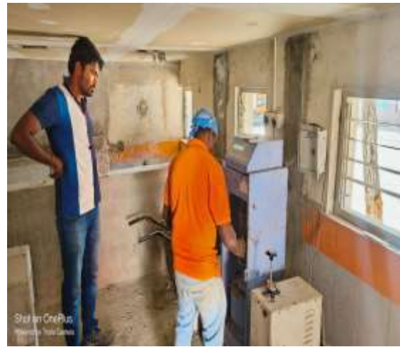
PCC Concrete Trial Mix Testing
