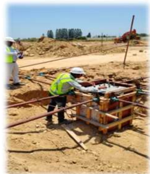
Anchor Bolt Fixing & Checking
