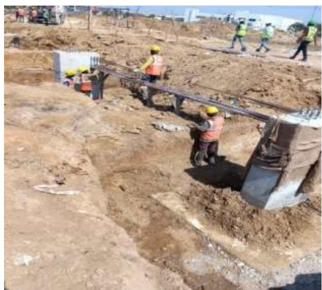
Plinth Beam Shuttering and Concrete Casting
